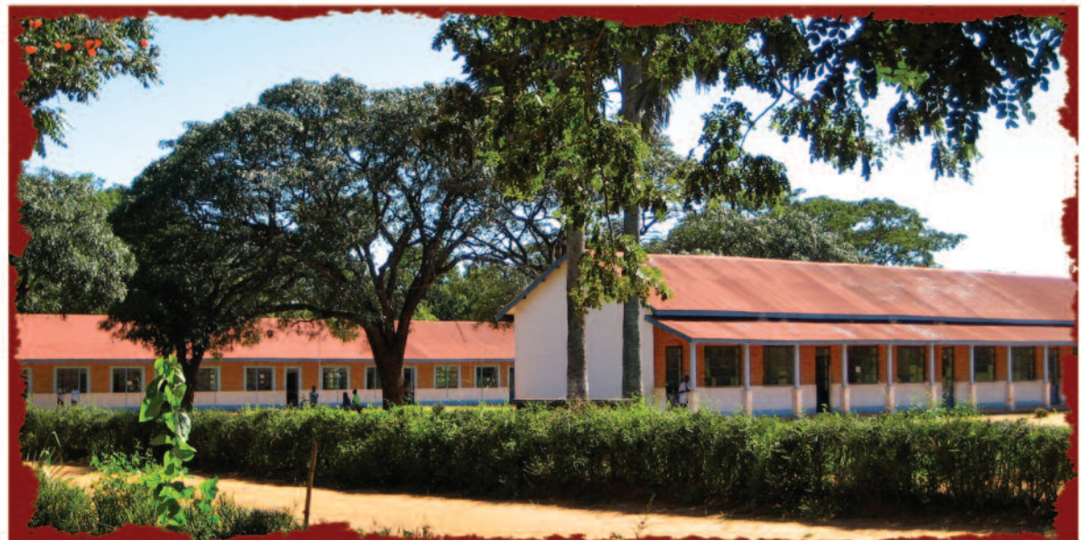
The dilapidated school buildings are slowly coming back to life now that our Brothers are once again a presence.
